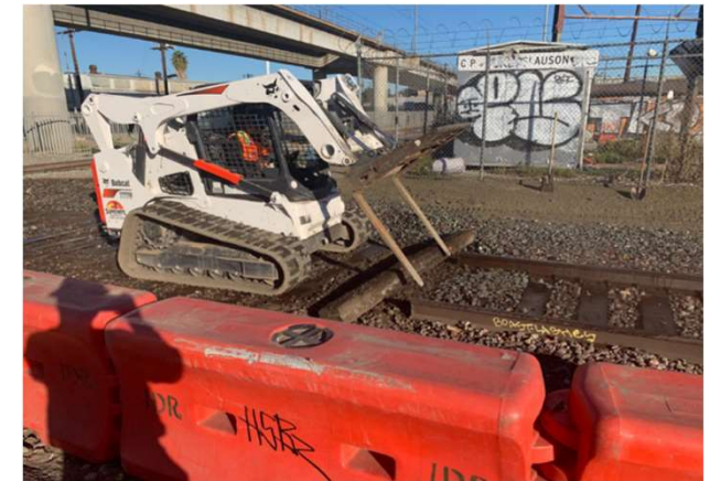
Removing ties for load out
