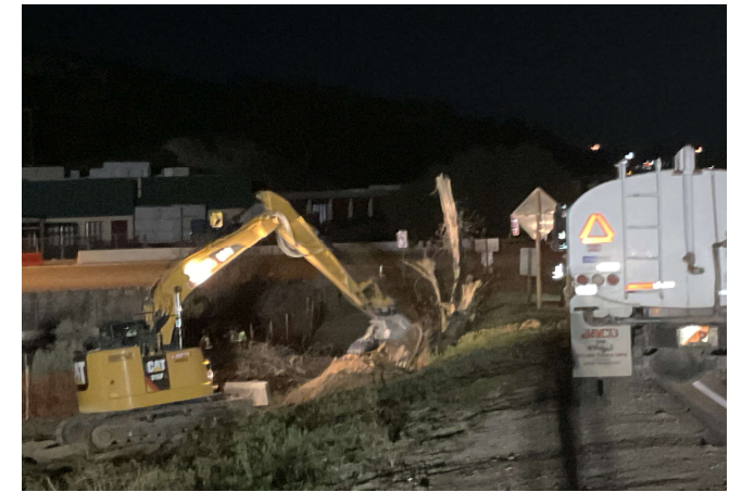
I-5-SB / Cal-Grove Blvd on-ramp clearing and grubbing work in progress
