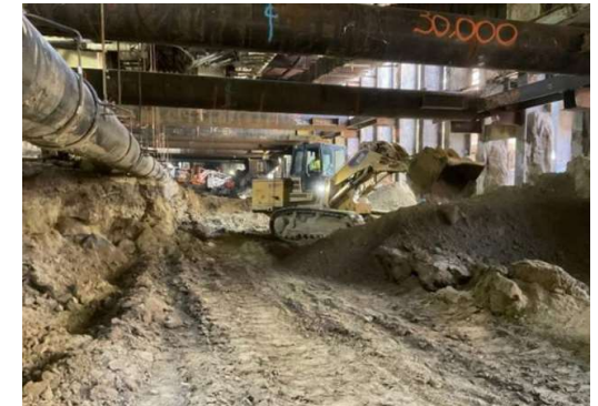
Century City Constellation Station Box Excavation
