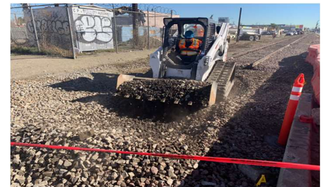
Sorting ballast on the east side of the UPRR track
