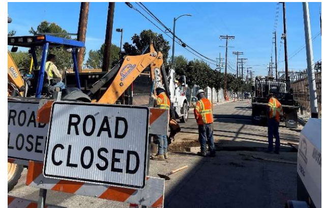
DWP Sylmar Undergrounding
