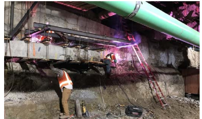
Utility support installation for DWP Power and Storm Drain Box on Flower St
