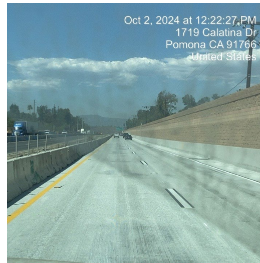
NB-71, completed stage 1 roadway.
