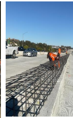
Median Barrier Rebar Installation
