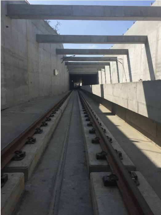
UG-1 - Tunnel section without the cover
