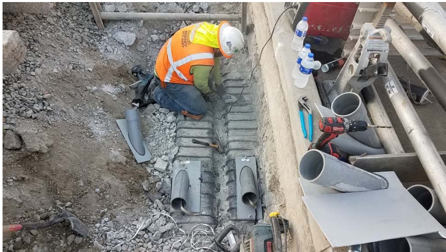
Modifying Existing Duct Bank
