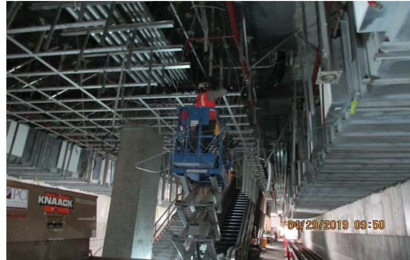
Installation of metal ceiling grid at the Leimert Park Station platform
