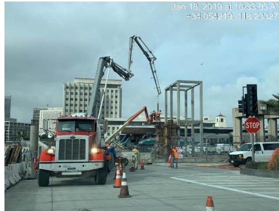
Pouring columns for the elevator structure
