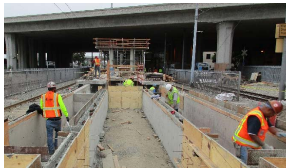
Formwork for south extension of Blue Line Platform
