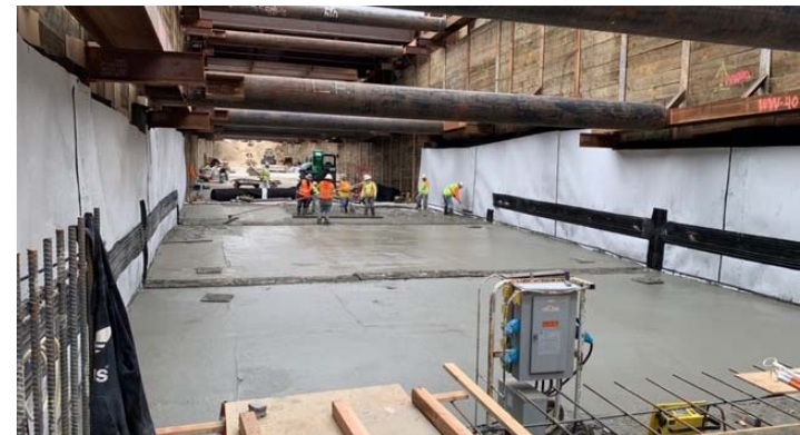
Protection slab placement at 1st Street Leg
