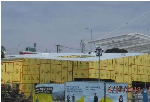
Exterior sheathing at Customer Service Building
