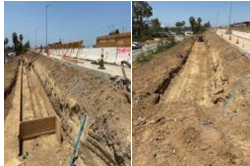
RW 245 Forming Footing
