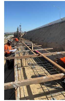
Retaining Wall 2809 Rebar Placement
