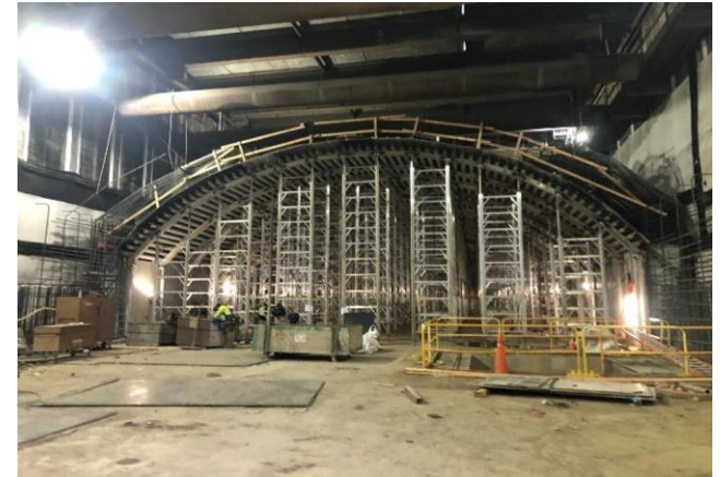
Westwood/UCLA Station: Falsework Supports for Roof Construction (Looking West)
