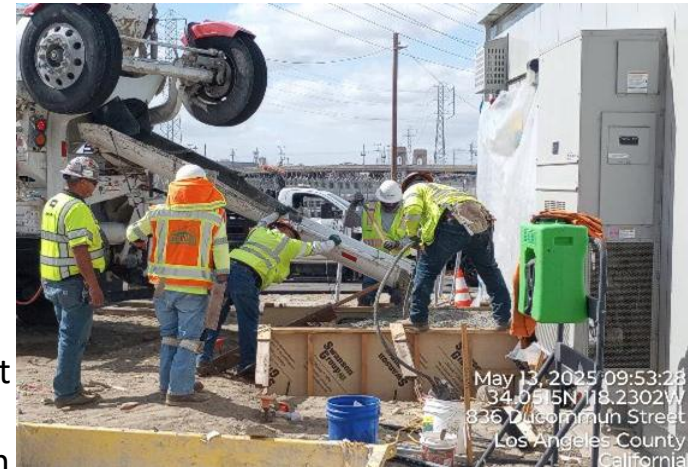
Placing concrete stairs and landings at the Portal Bungalow
