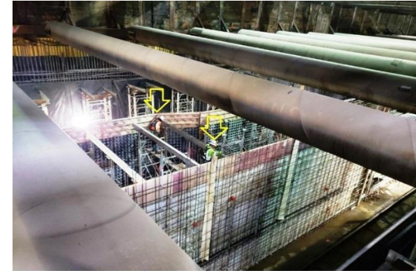
Wilshire/Fairfax Station Interior Wall Formwork
