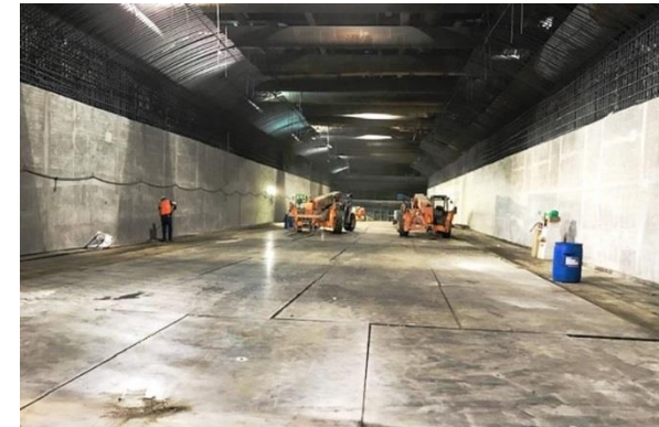
View of Wilshire/La Cienega Station Concourse Level
