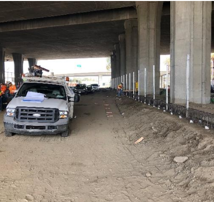
Grading Work @ Package B
