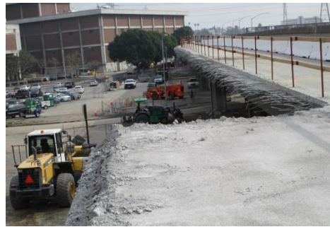
Edge of Deck Removal
