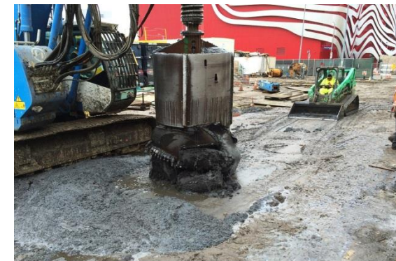
Drilling Piles near Wilshire and Fairfax
