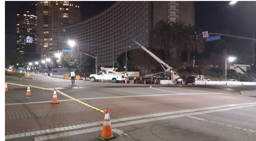
Telecom joint trench construction at Constellation Boulevard
