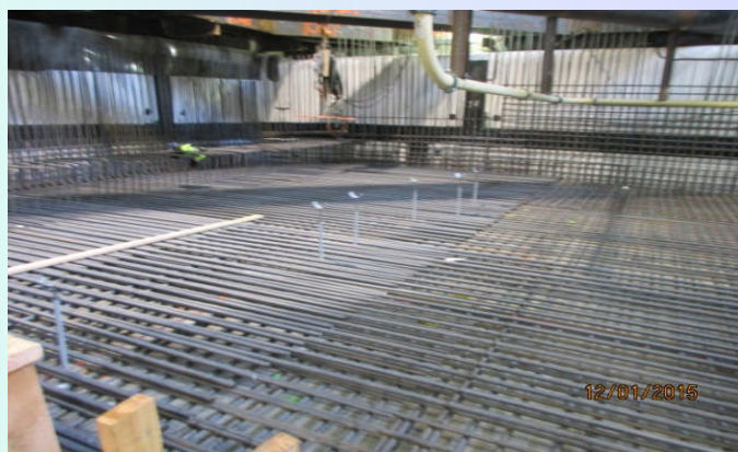
EXPO/CRENSHAW STATION – Installation of rebar for invert slab placement.
