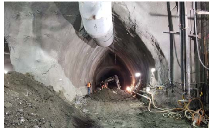
SEM Cavern right drift excavation
