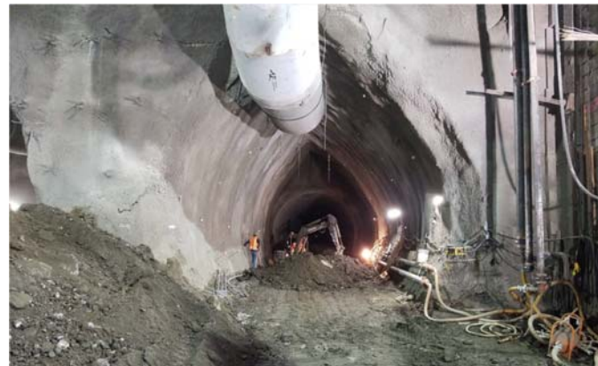
SEM Cavern right drift excavation
