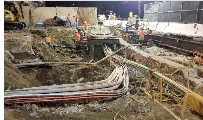
Utility work on Flower Street
