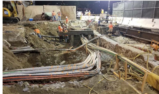
Utility work on Flower Street
