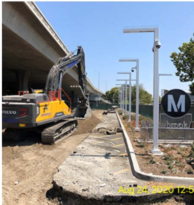
Grading Work @ Package B
