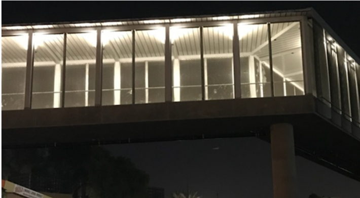
Pedestrian Overcrossing to Patsaouras Bus Plaza
