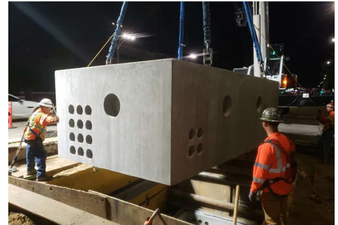
Installation of 1 of 4 vaults by on Van Nuys Blvd, between Vanowen and Vose.
