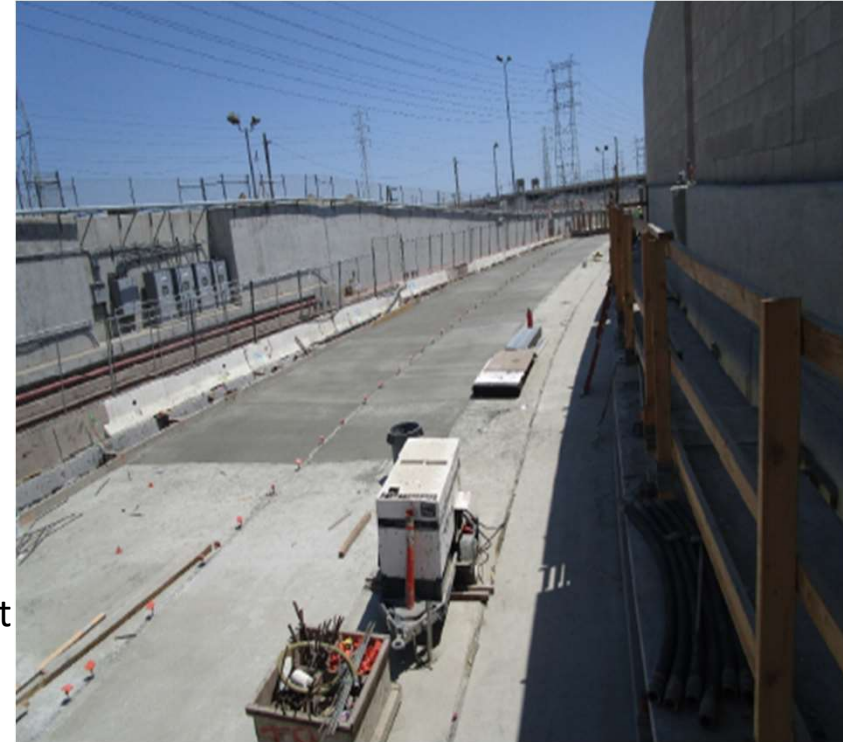
Portal –West Retaining Wall and invert
