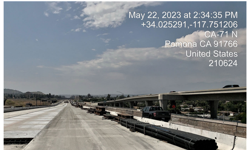
JPCP paving in the median
