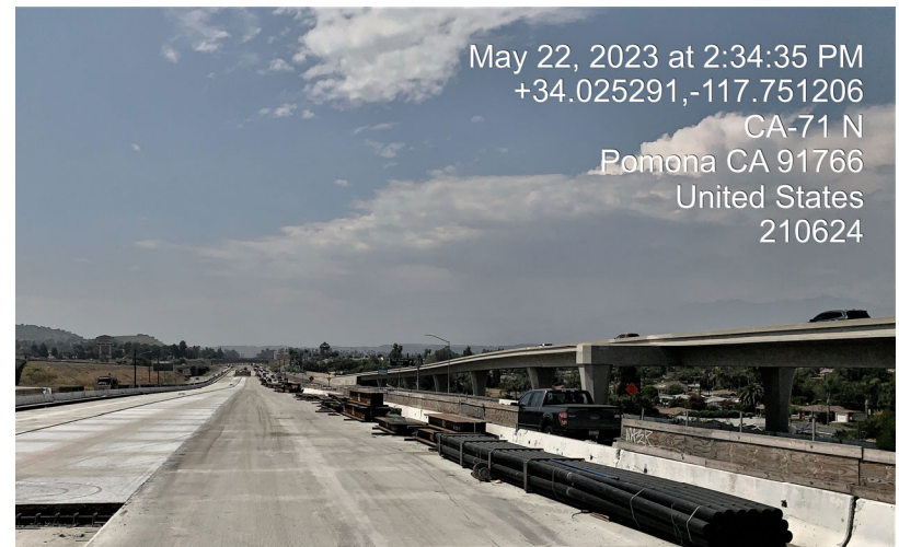
JPCP paving in the median
