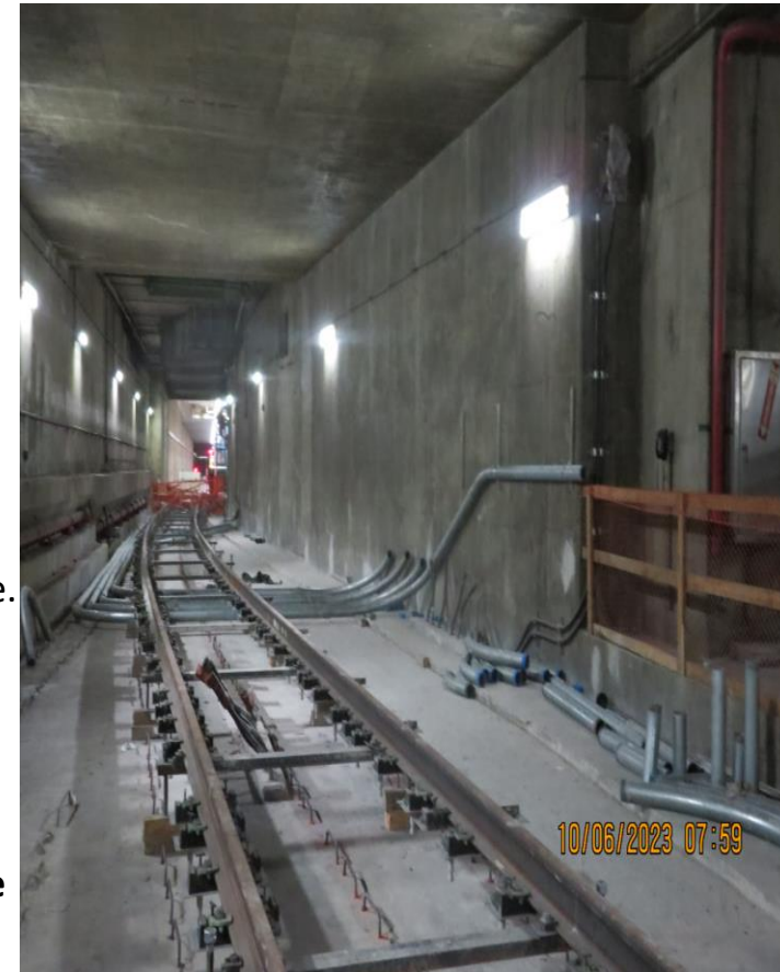
East Union Track Placement
