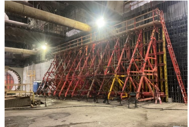
Century City Constellation Station - Concrete Placement
