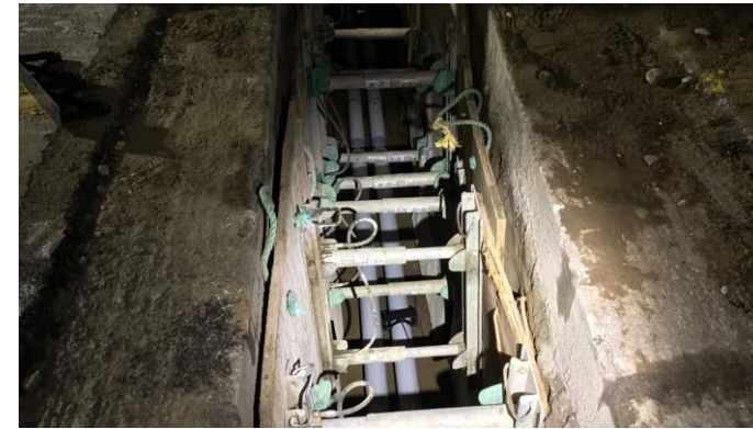
C1220 Ductbank Installation
