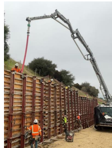
Pouring concrete at Retaining Wall 2461
