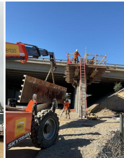
Forming and preparing to pour Rye Canyon bridge bent cap
