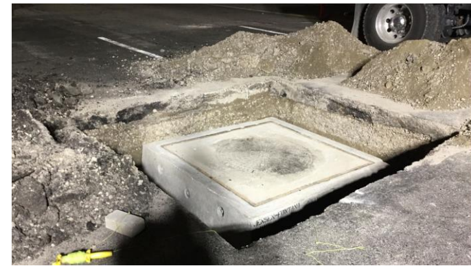
C1220 Manhole Installation
