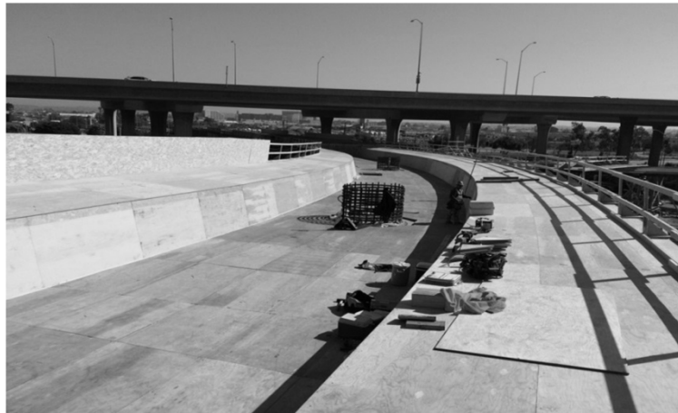
Green Line tie-in formwork placement continues over Aviation Blvd.
