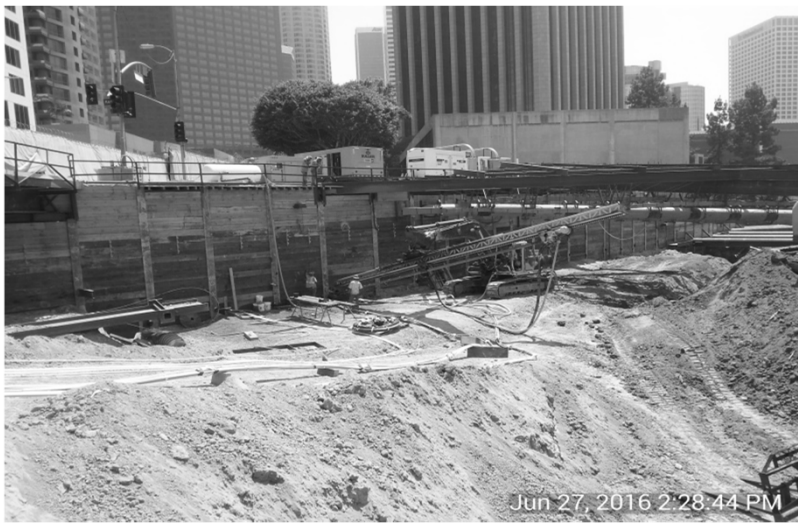
Structural excavation at 2 nd /Hope
