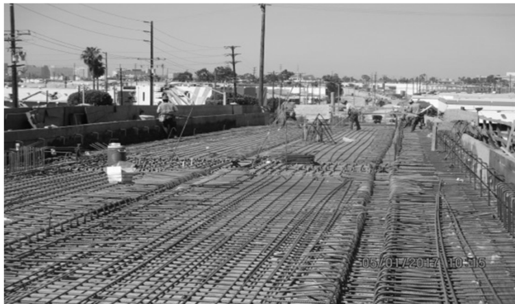
Preparing for a deck pour on the I-405 bridge structure.
