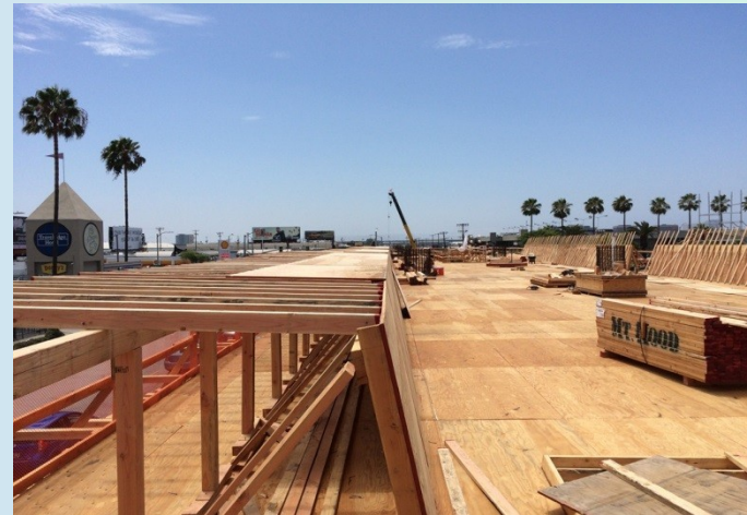
AVIATION/CENTURY STATION – Bridge falsework for concrete pour
