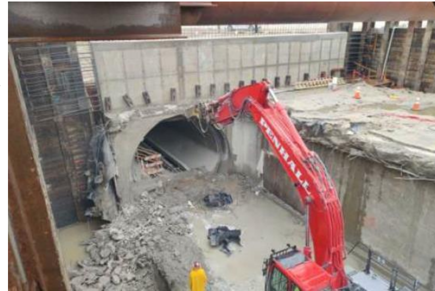
West Portal Wall Demolition
