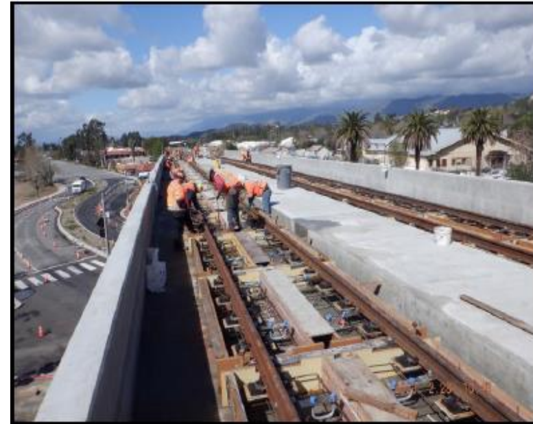
Bonita / Cataract – Structure Track Direct fixation
