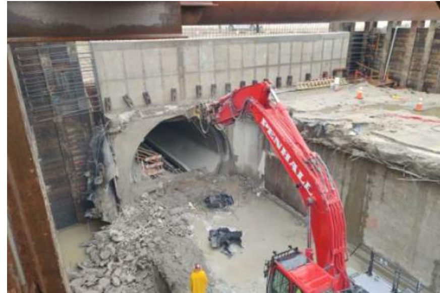
West Portal Wall Demolition
