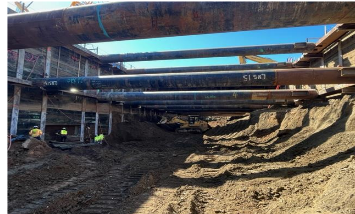
Westwood/VA Station: Excavating station for Level 2 Bracing
