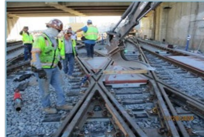
Crossing Panel Installation
