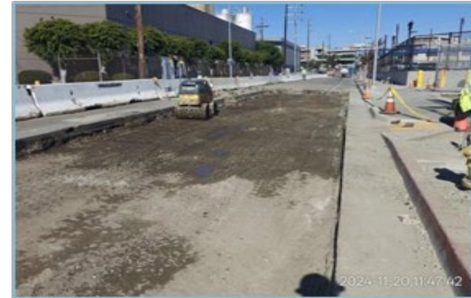
Center Street Reconstruction
