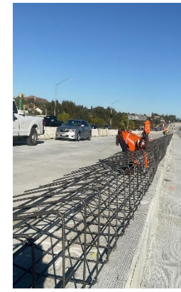
Median Barrier Rebar Installation
