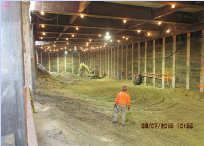
LEIMERT PARK STATION – Excavation and lagging
