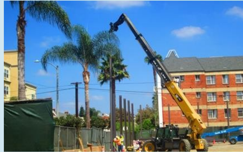
Soundwall Construction at North Wilshire/La Brea
