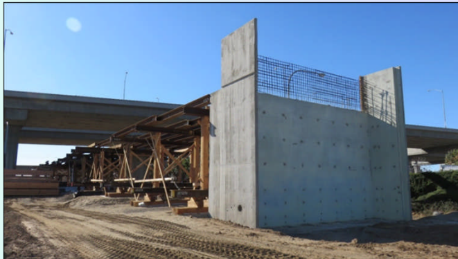
Greenline bridge falsework construction ongoing
