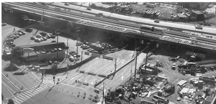
Aerial view of site
