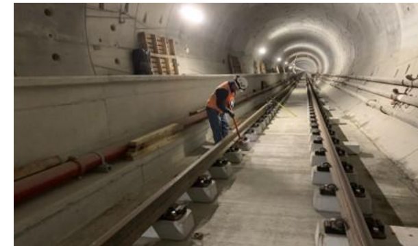
Reach 1 Track Installation
