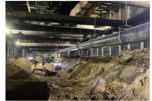
Century City Constellation Station Box Excavation
