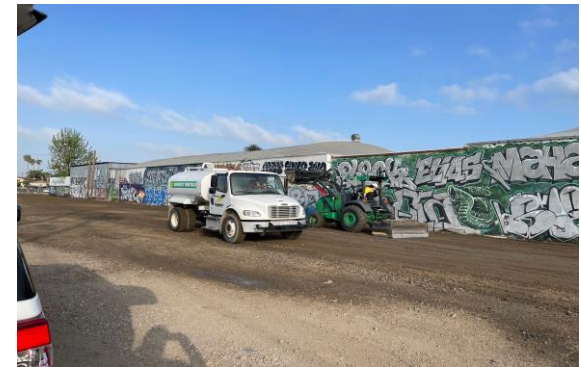
Site preparation work
