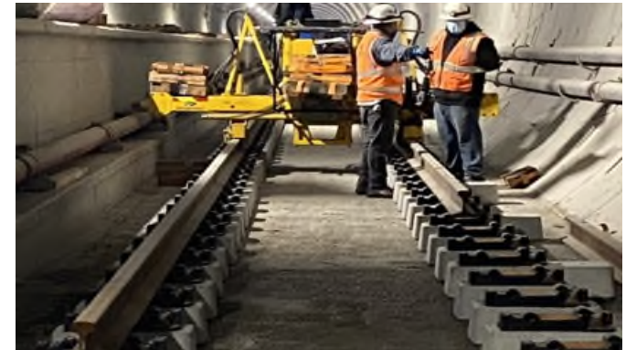
Track Installation in the Reach 1 Tunnel
