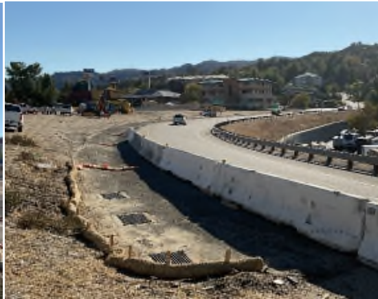
Placement of temporary work zone speed radar and stormwater pollution prevention materials
