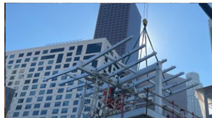
Canopy installation at Grand Av Arts/Bunker Hill Station
