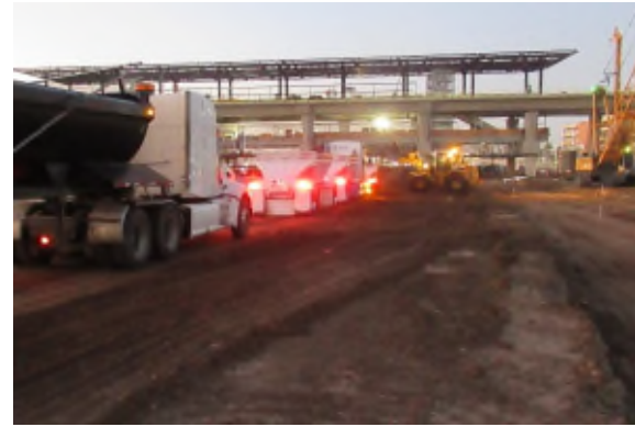
Early morning soil removal work
