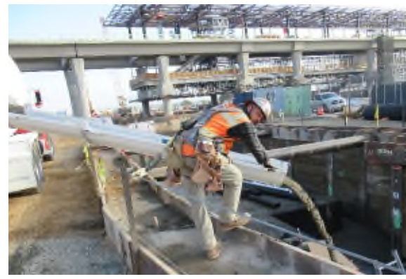
Backfill at cisterns
