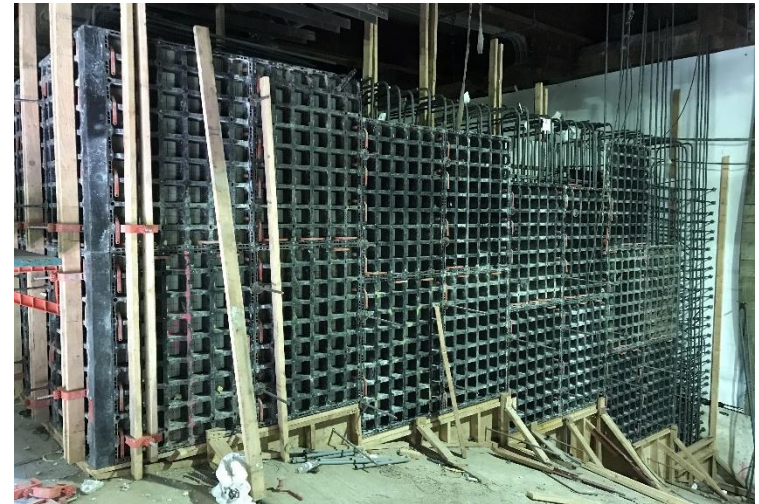
Wilshire Rodeo Station East EVS Shaft-East of Station-Rebar and Formwork
