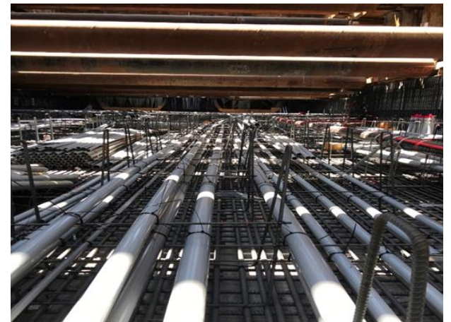
Westwood/VA Hospital Station: Traction Power Conduit Install (Looking West)
