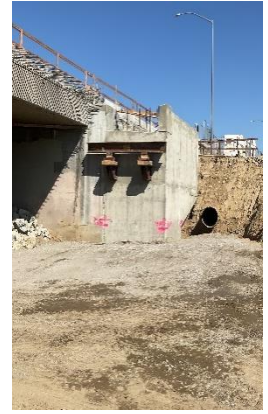
Castaic Creek Bridge Abutment 4 Complete
