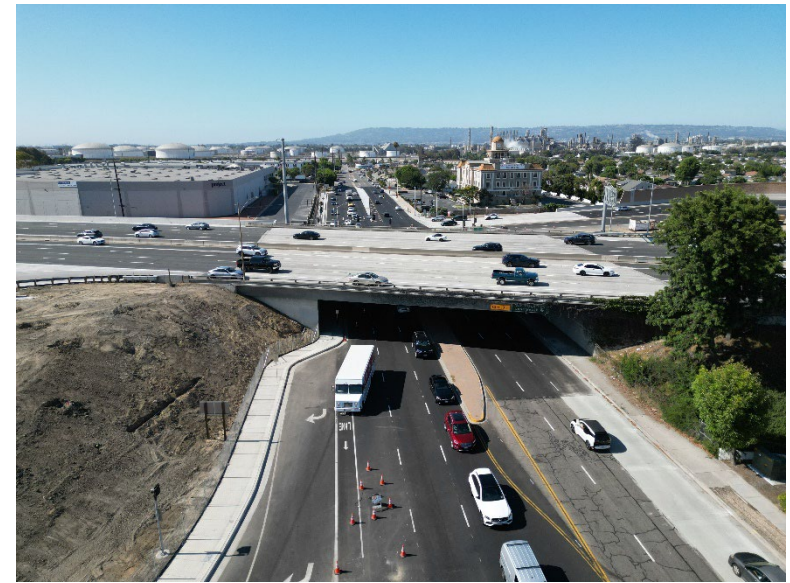
North side of Crenshaw Blvd UC (Looking South) showing Crenshaw Blvd improvements/auxiliary lane for new NB loop ramp.
