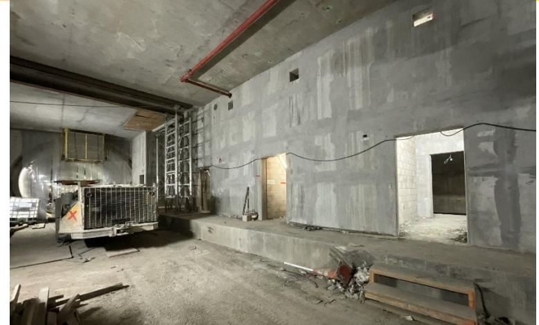
Century City Station CMU walls on Rooms at Track Level Crossover
