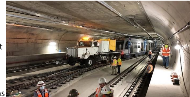
Dead pull test in Crossover Cavern
