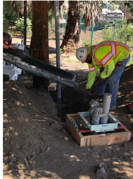
Pilot Gate - DWP Service Pedestal Installation
