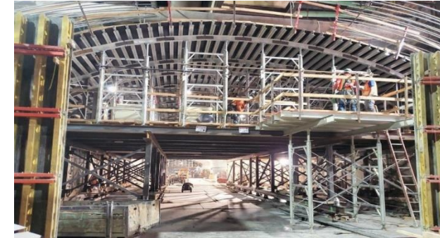
Roof Falsework Installation at Wilshire/Fairfax Station
