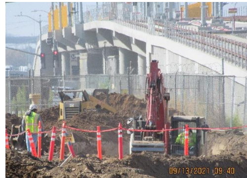
Backfill Work at South End of Site
