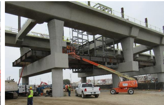
LAVA APM Steel Work in Progress
