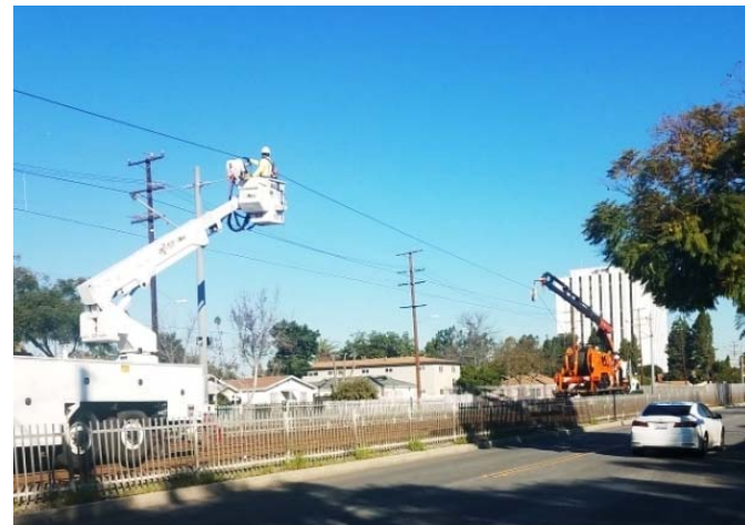
Overhead Catenary System Demolition
