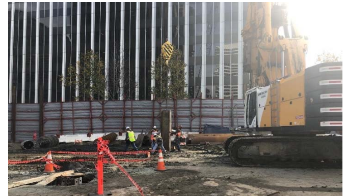
Soldier Pile Installation in Century City
