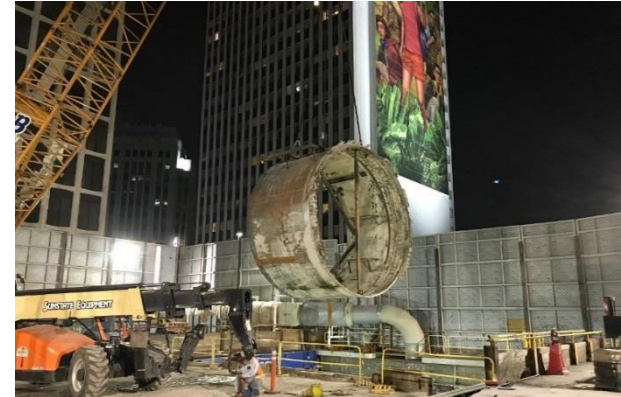
TBM Gantry Shield at Wilshire/Western
