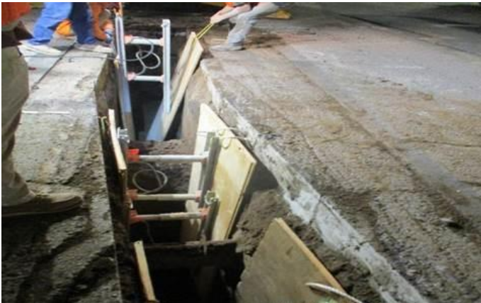
Hand Dug Excavation for Fiber Optic Conduit
