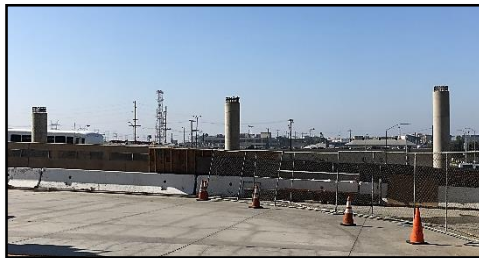
Pedestrian Walkway Columns
