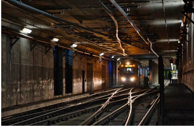
Testing of the new Overhead Conductor Rail (OCR)
