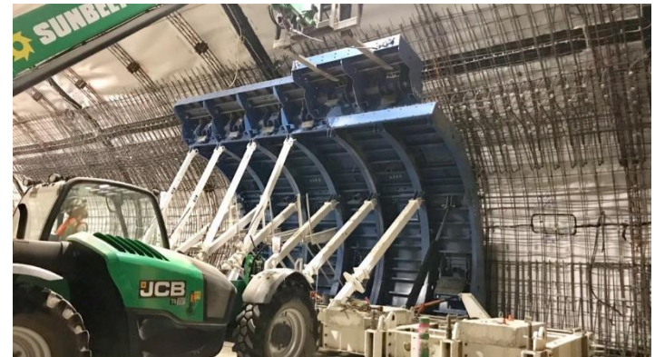
Wall form installation in SEM Cavern
