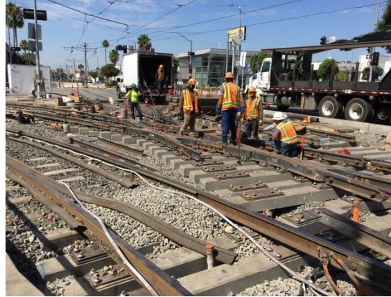
Replacing trackwork at Expo Junction
