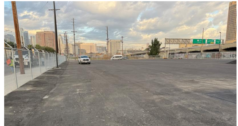
Life Storage demolition and paving completed November 2025
