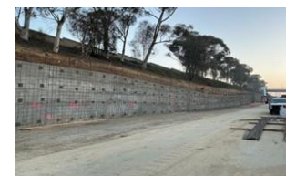
105WB RW 270 Soil Nail Wall Exterior
