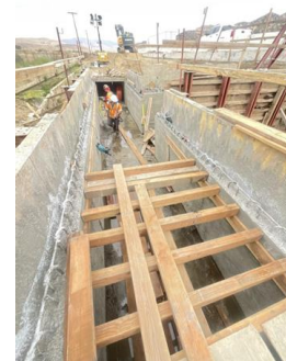
Drain System 406 Formwork Install
