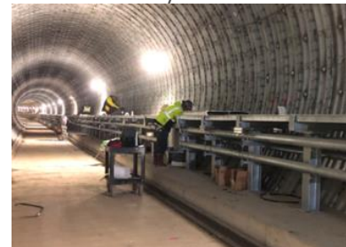
Tunnels: Steel Walkway Construction BL Tunnel
