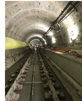
BL R4 Completed Second Stage Invert Track Concrete Pour
