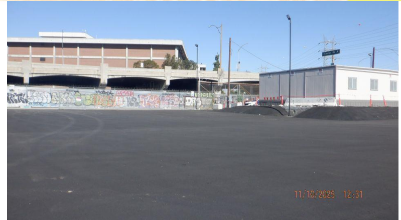
Life Storage demolition and paving completed November 2025
