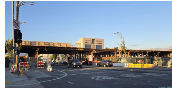
Falsework for Van Nuys Bridge
