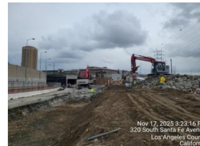
East Portal Demolition
