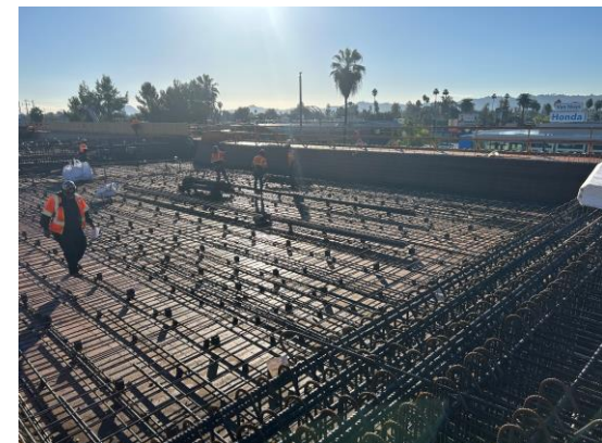
Rebar Installation at Van Nuys Bridge
