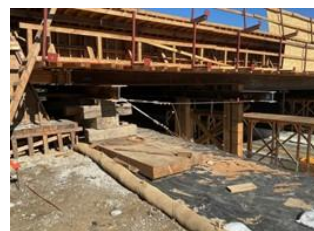
105EB stanford bridge falsework
