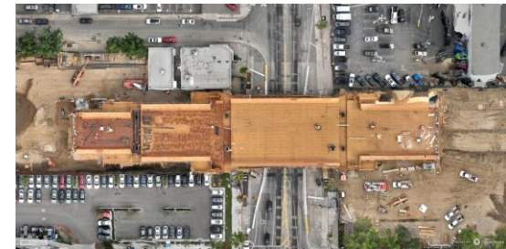
Aerial View of Van Nuys Bridge Construction
