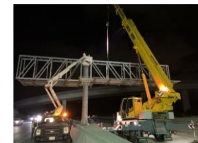
Sign Structure Truss Installation
