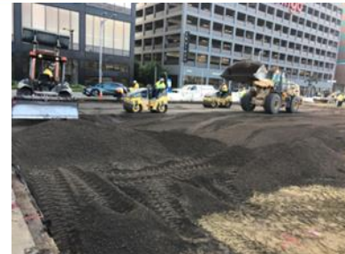
Westwood/UCLA Station: UCLA Main Station Box Backfill on Wilshire Blvd
