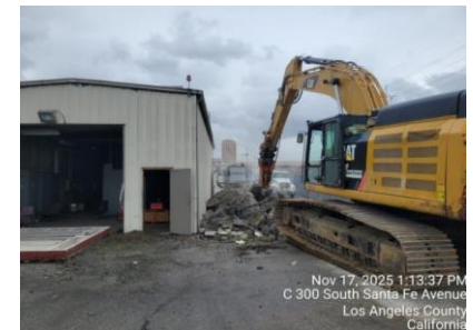
Legacy TPSS Demolition
