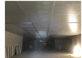
CCS - West Upper Concourse Installation of Metal Ceiling Panels
