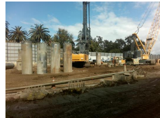
Pile Installation for TTES
