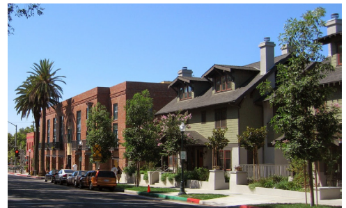
Figure 28 Residential transition at Mission Meridian Village, a transit oriented development along the Gold Line in Pasadena.
