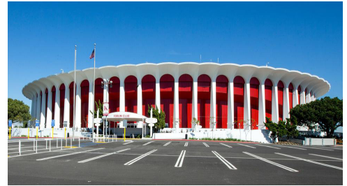
Figure 6 The Forum, located at 3900 West Manchester Boulevard in the City of Inglewood.
