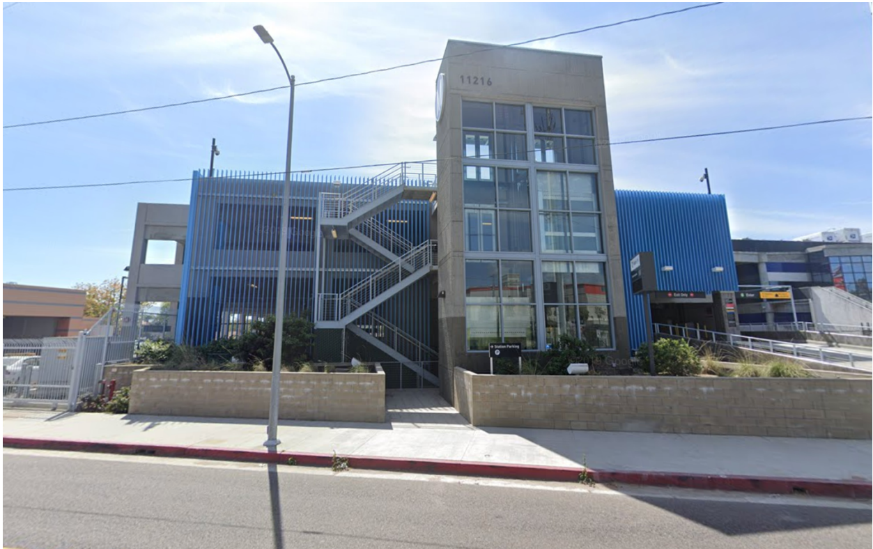
Figure 4.10.9 Expo/Sepulveda Parking Garage (view from Exposition Boulevard)
