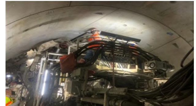
Ring Installation in the BL Tunnel
