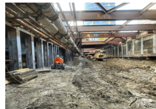
Constellation Station Entrance Excavation
