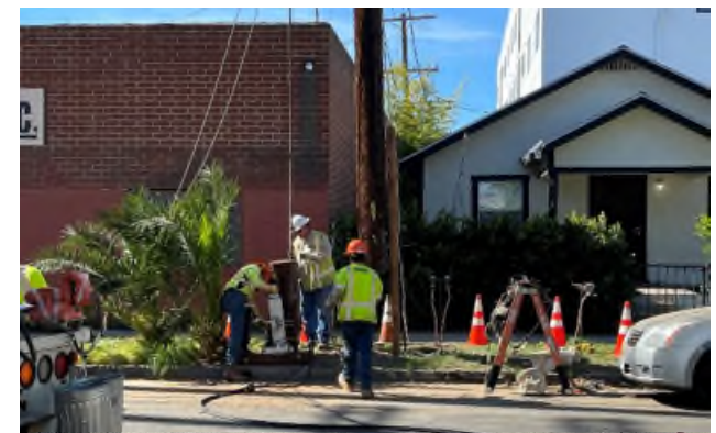
DWP Vesper Advanced Utility Relocation
