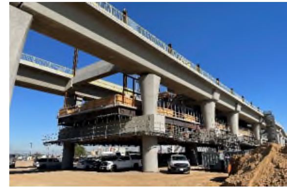
LAWA Station work in progress
