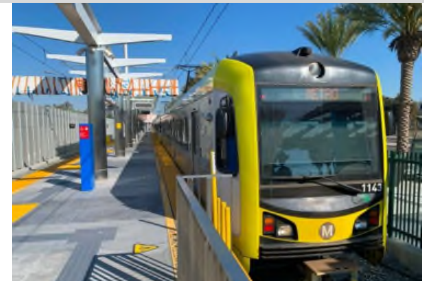
Downtown Inglewood Station – Train testing
