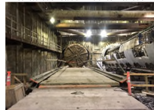
Ruth Breakthrough at Wilshire/Rodeo Station
