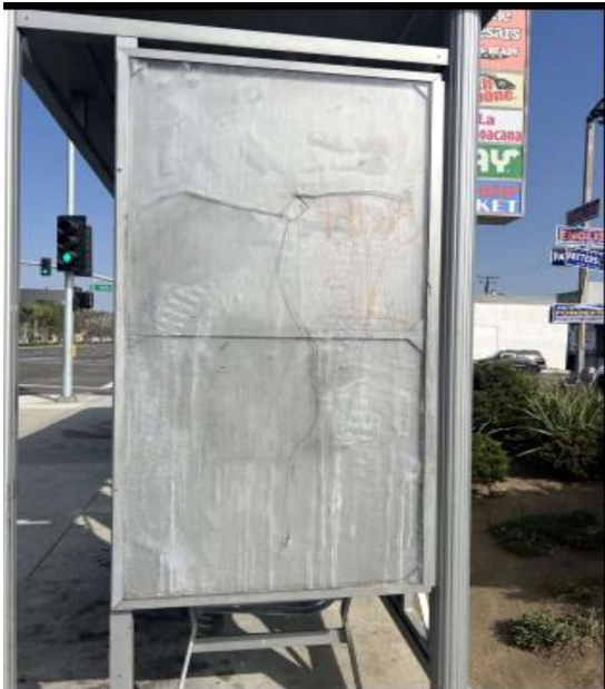
Picture 11 - Hawthorne & 118 th (Broken Plexiglass)
