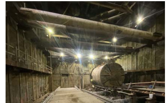
Harriet Breakthrough at Wilshire/Rodeo Station
