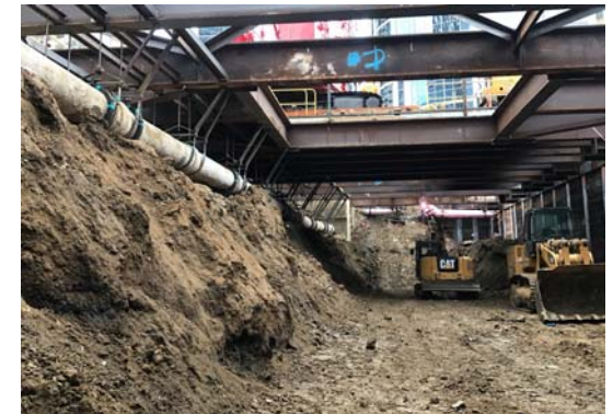
Constellation Station Entrance Excavation
