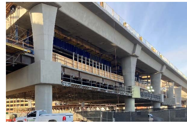
LAWA Station work in progress
