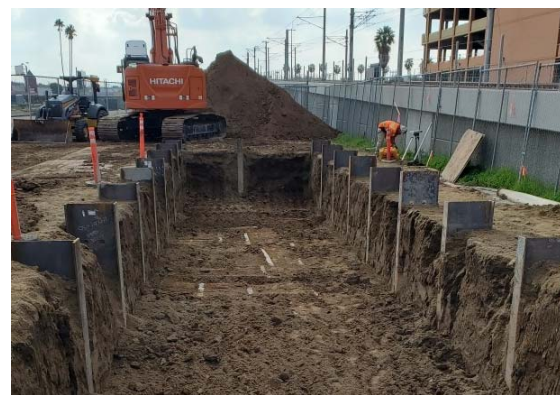
Shoring in progress
