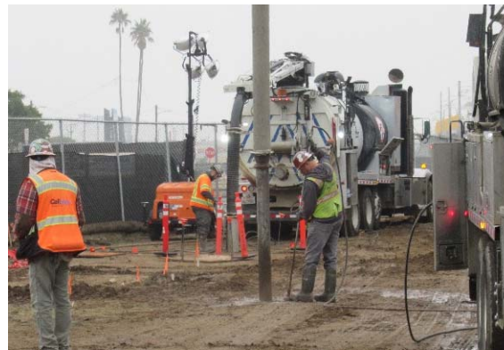
Shoring installation for Stormwater System
