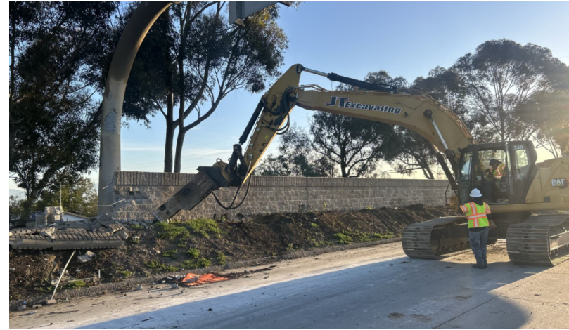
Clearing and Grubbing with removal of the existing sound walls
