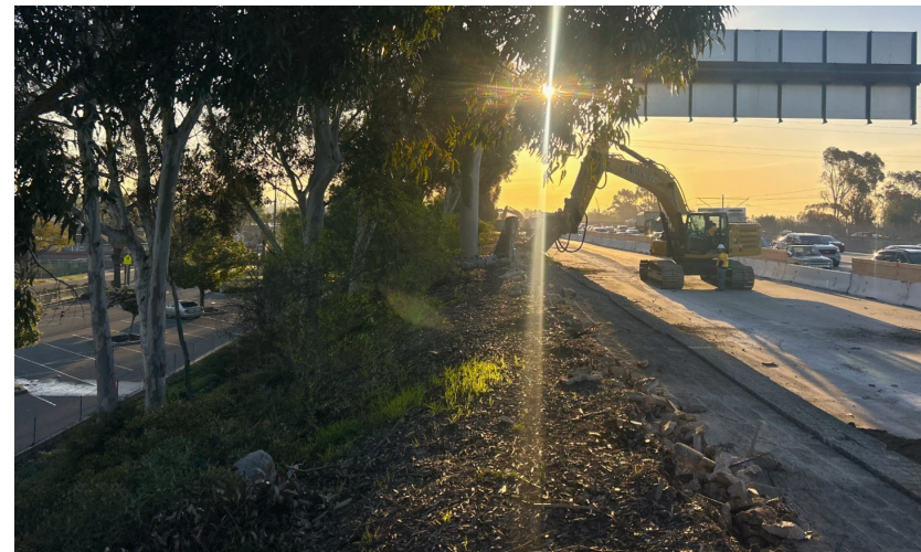
Clearing and Grubbing with removal of the existing sound walls
