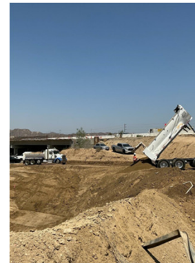
Embankment Fill at Rye Canyon
