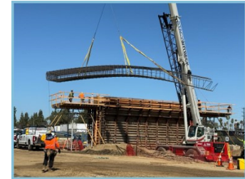
Setting Reinforcing Steel at Van Nuys Abutment 5
