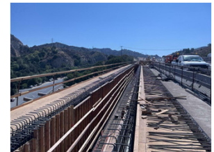
Gavin Canyon Bridge Right Formwork
