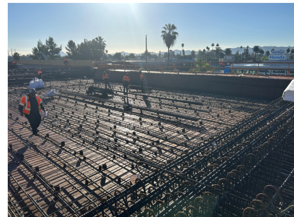
Rebar Installation at Van Nuys Bridge
