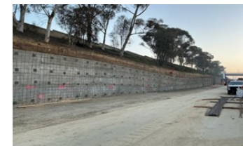
105WB RW 270 Soil Nail Wall Exterior
