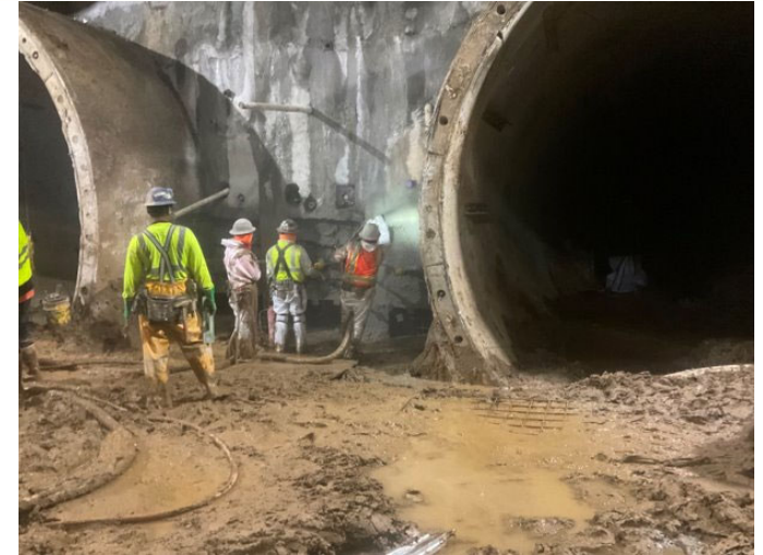
Westwood/UCLA Station: Placing Shotcrete for Row 4 Soil Nails at East Headwall
