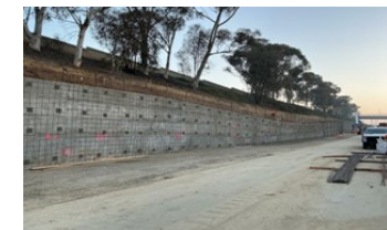
105WB RW 270 Soil Nail Wall Exterior
