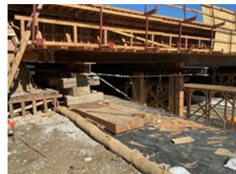
105EB Stanford bridge falsework
