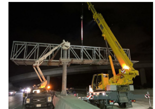
Sign Structure Truss Installation
