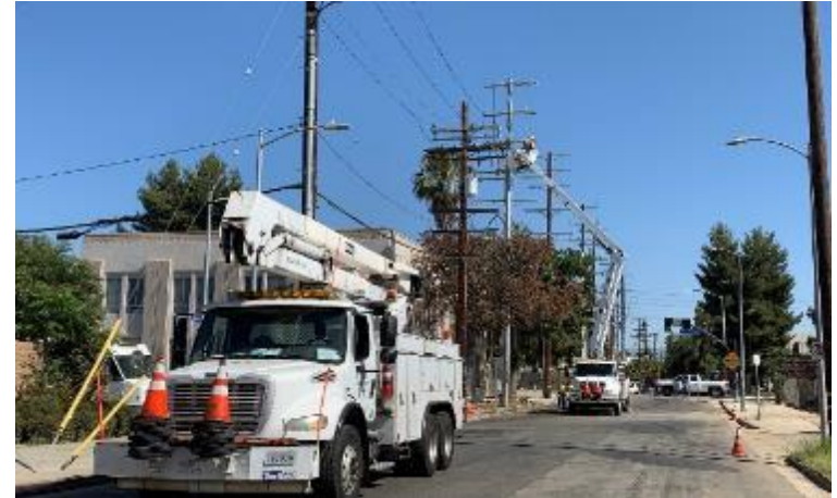
DWP Overhead Construction at Vesper
