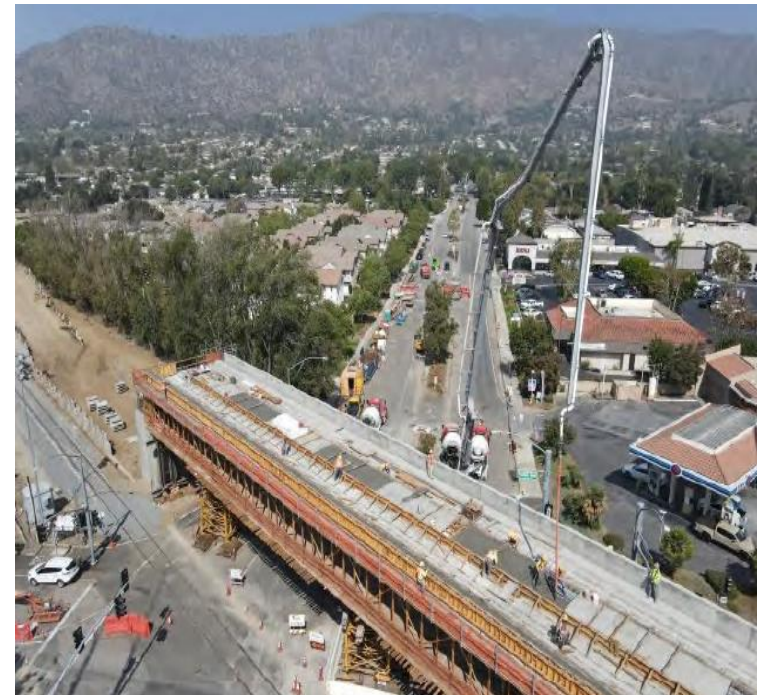
Foothill Grand - LRT ductbank walkway
