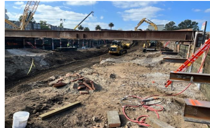
Westwood/VA Station: Excavating station to Level 1 Bracing
