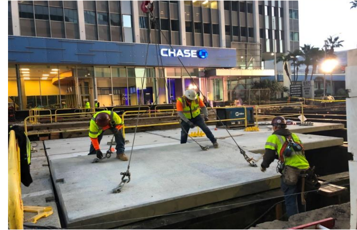
Westwood/UCLA Station: Installing Temporary Deck Panels in Wilshire Blvd
