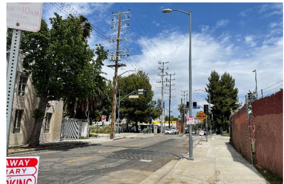
DWP Overhead Construction at Vesper
