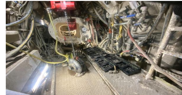
BR TBM – Hyperbaric Intervention Cutting Tool Replacement
