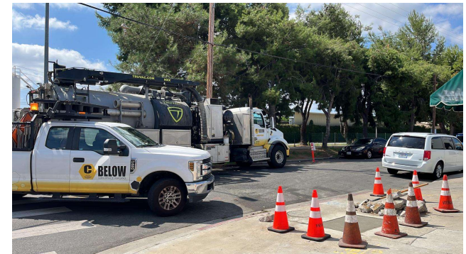
Sidewalk Panel Restoration on Bessemer St
