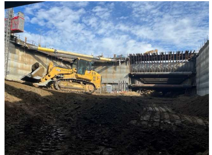
Westwood/VA Hospital Station: Excavation for Level 4 Support
