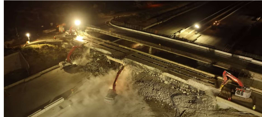
Demolition of old Weldon Canyon Bridge
