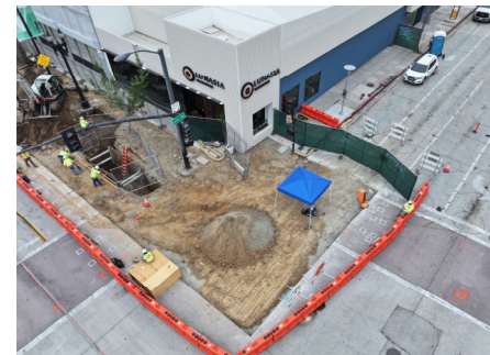
Colorado and Lake Westbound Station Construction
