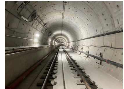
Tunnels: Completed Running Rail Installation
