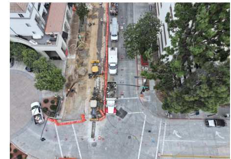
Holly and Arroyo Westbound Station Construction
