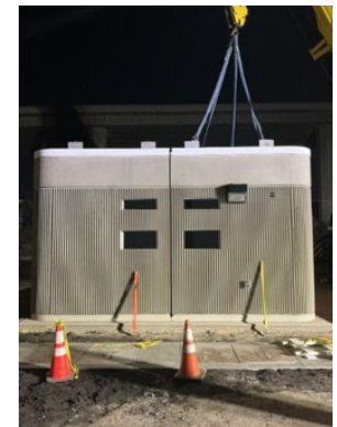
Setting of HUB Building
