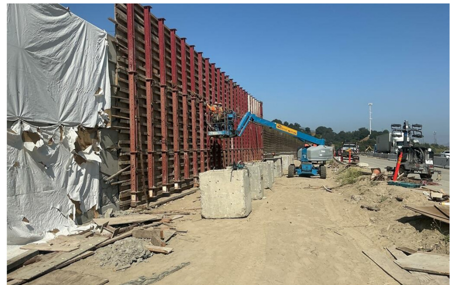
Retaining Wall 2449 Formwork Installation
