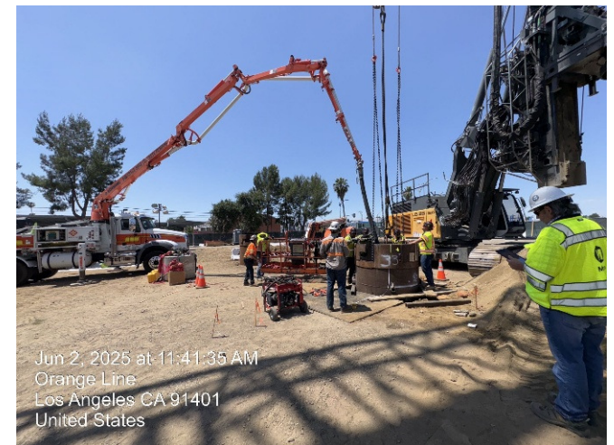
CIDH Foundation Installation at Van Nuys
