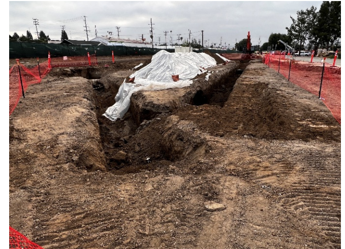
Storm Drain Removal at Van Nuys
