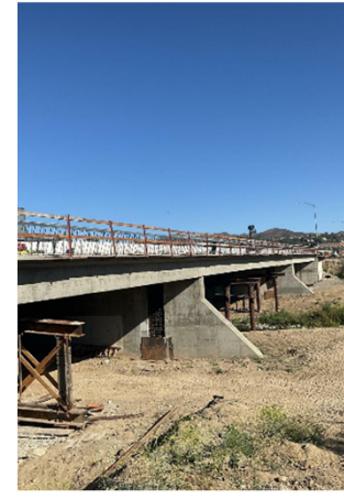
Castaic Creek Bridge Falsework Lowering
