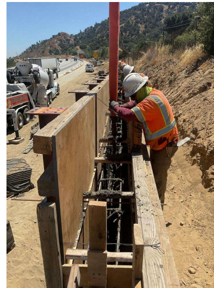
Pouring concrete at Retaining Wall 2461
