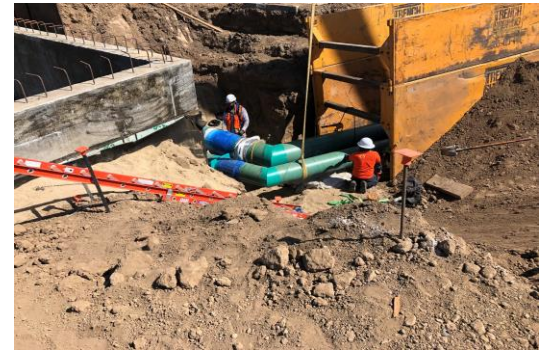
VA Steam Tunnel: Installing Redundant System (Condensate and Steam Line)
