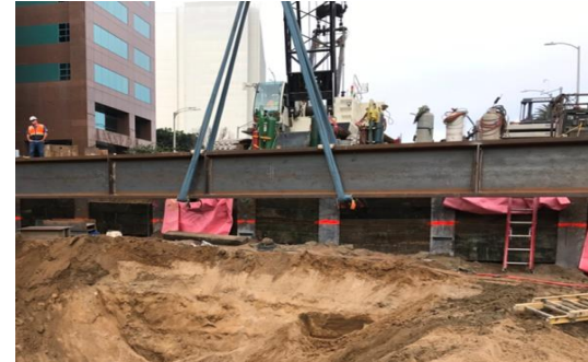
UCLA Station: Installing Structural Steel Beams for Temporary Decking
