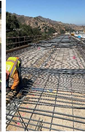
Gavin Canyon Bridge Deck Rebar Install
