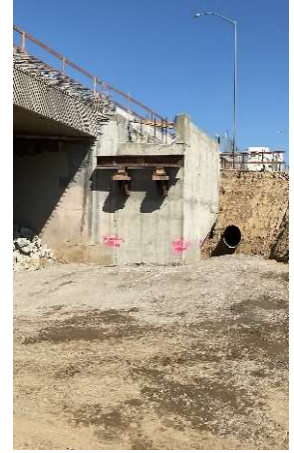
Castaic Creek Bridge Abutment 4 Complete
