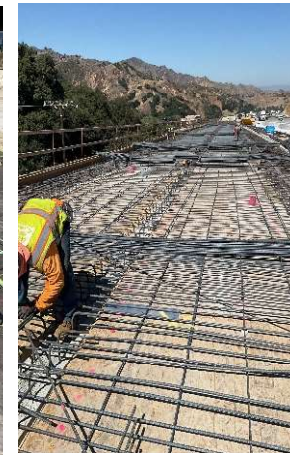
Gavin Canyon Bridge Deck Rebar Install
