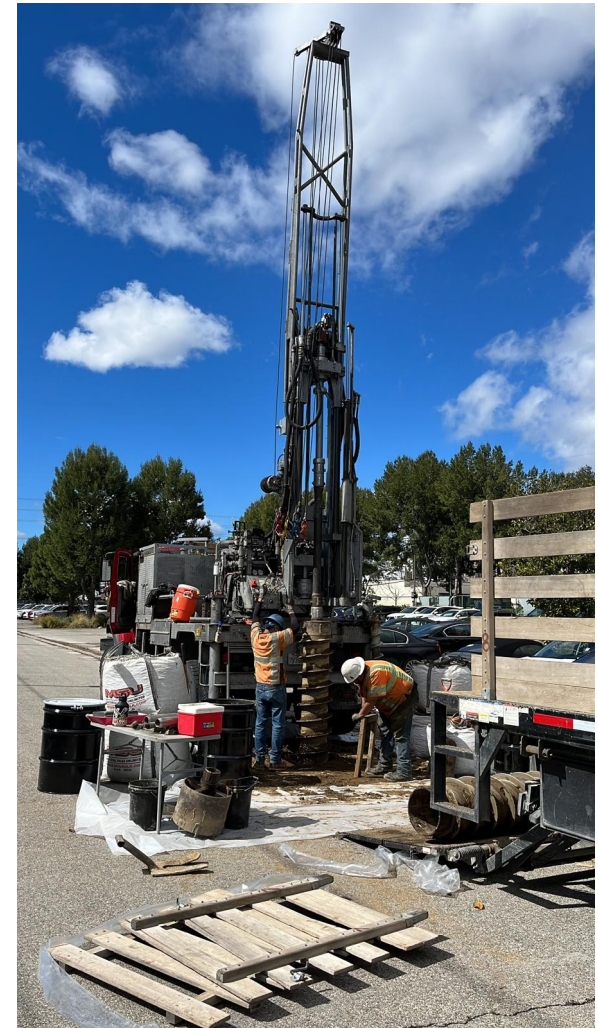
Geotech- percolation testing for stormwater capture scope
