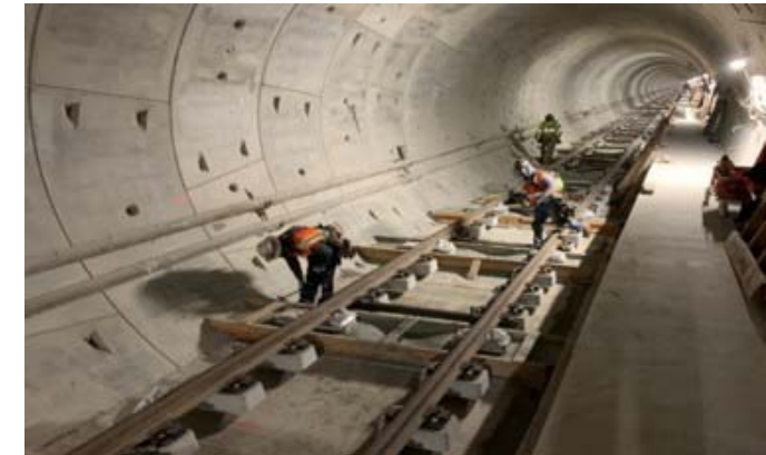
Reach 1 North Tunnel Trackwork Installation
