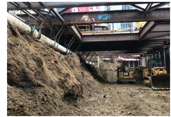
Constellation Station Entrance Excavation
