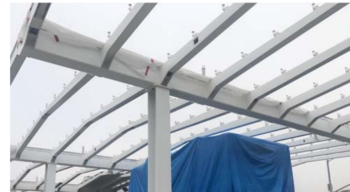
Little Tokyo/Arts District Station Canopy Installation
