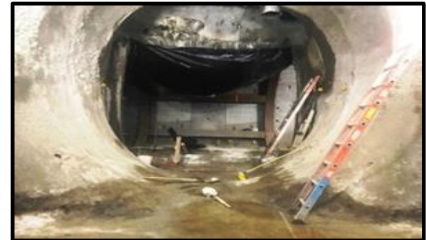
View of Reach 1 Cross Passage #8
